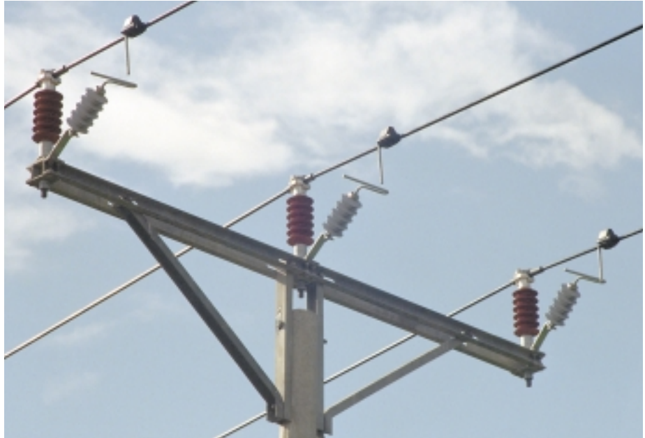
Covered conductor system protected by CLX
