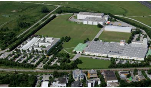
Energy headquarters Munich/Germany
