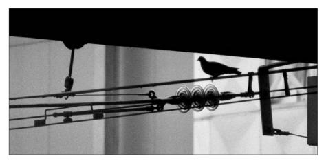
Electrical failures frequently result when birds perched on catenary wires make contact with the bridge as they fly away to avoid oncoming trains. This problem is overcome by insulating the catenary wires with Raychem FCSM tubing as shown here
